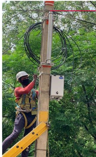
Utility Pole ready with Mount and Enclosures
